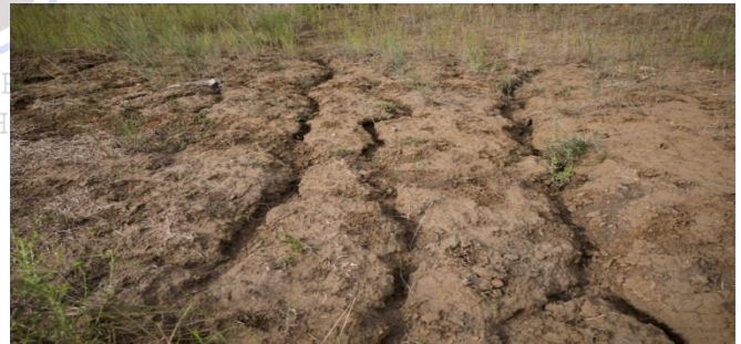
Channels created by rill erosion
